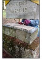
Wet the stone surfaces thoroughly before applying the mortar and sponge off any excess water. You want the stone to be moist so that it does not suck the water out of the mortar. Apply the mortar in a thin, even layer covering the entire contact surface on the lower stone with the edge areas slightly higher. Painters tape can be used to prevent excess mortar from getting on
