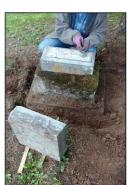
Do not use concrete, do not use any off-the-shelf mortars, all are too hard. You need the softness of lime mortar to prevent damage to the stone. The mortar joint has to be the weak link on a monument so that if the headstone does get pushed over in the future, the mortar joint will be the first to fail.
