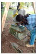
For resetting a stone on a base or plinth, the rule is to use 1 part natural hydraulic lime (NHL 3.5) to 2 parts clean fine sand. For resetting a stone in a base slot, the rule is to use 1 part natural hydraulic lime (NHL 3.5) to 3 parts clean fine sand. Stir the dry ingredients, adding small amounts of water until damp. Stir for about 8 minutes, and the lime mortar will become slaked and be the consistency of peanut butter. The mortar should remain workable for about 30 minutes.
